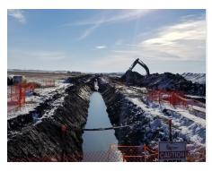
Description & Location: SF25 Facing East Excavator loading rock truck Water in trench
