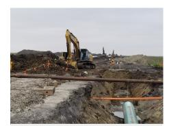
Description & Location: SF5 Facing West Excavator digging trench while caterpillar moves clay to side.
