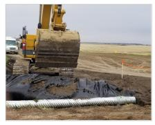
Description & Location: SF3 Facing West Excavator removing clay and Geo-tec from south half of approach.
